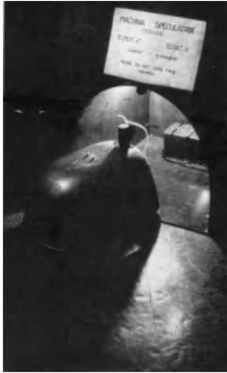
Fig. 2. One of the first model animals, Elsie, returns to the recharging station in her hutch. The notice reads “Machina speculatrix (Testudo). Habitat: W. England. Please do not feed these machines.” This picture, from an unknown source, dates from 1949.
